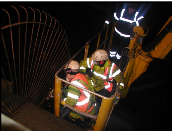
Removal of anti-vandal Guards
