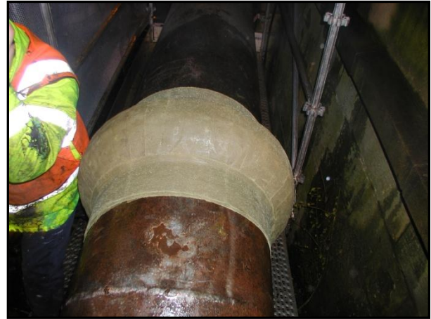
Pipe joint profiled and wrapped
