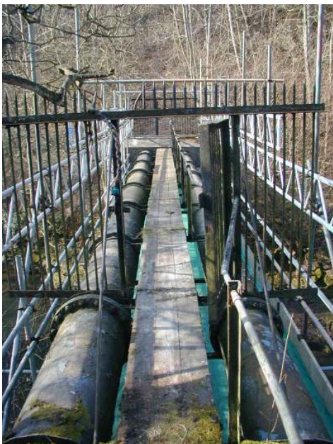
PIPE CROSSING FOOTPATH PRIOR TO RECOATING
